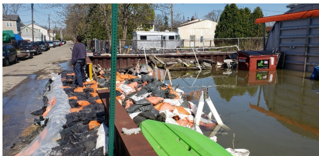
Figure 16: Sandbagged property in Jefferson-Chalmers community, Detroit, MI, May 2019
