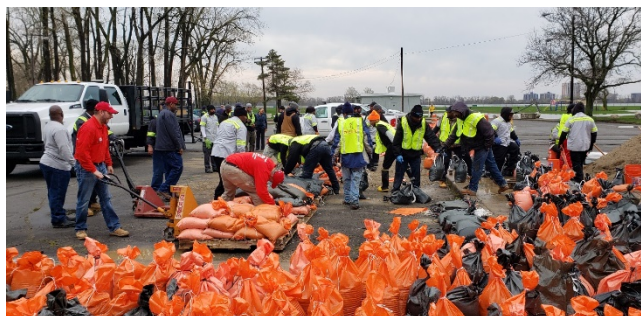
Figure 15: Flood Fighting Staging Area in Jefferson-Chalmers community, Detroit, MI, May 2019
