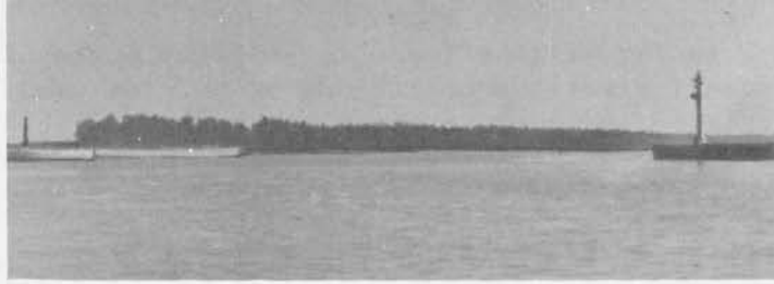
Port Weller Entrance
