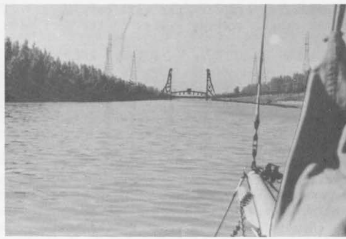
One of the 21 bridges in The Welland Canal.
