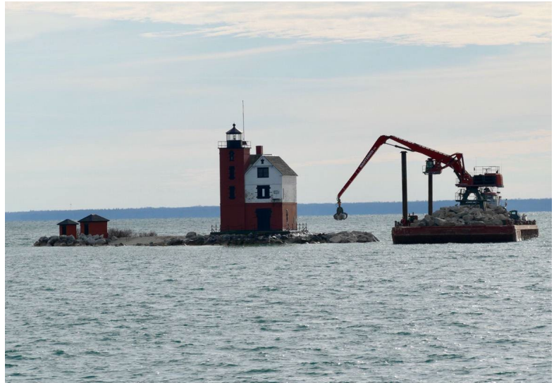
Contractor, North Shore Marine Terminal out of Escanaba, MI places rock around Round Island Lighthouse. Photo courtesy of Keepers of Round Island Lighthouse.
