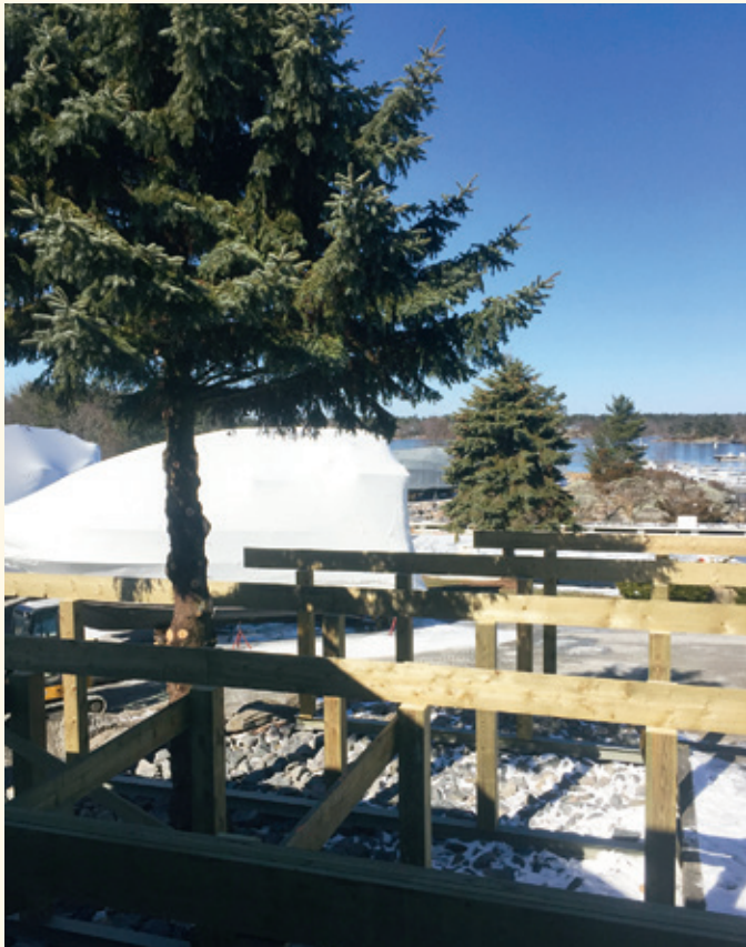
The new upper deck under construction.
